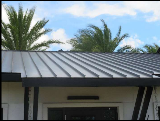
Clubhouse metal roof
