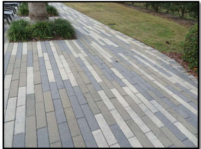
Masonry paver pool deck
