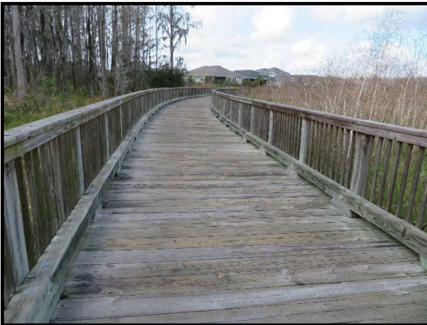
Boardwalk behind homes at Satilla Loop and Aviles Parkway
