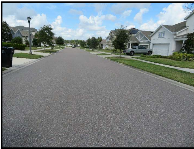
Asphalt pavement at Renaissance Avenue
