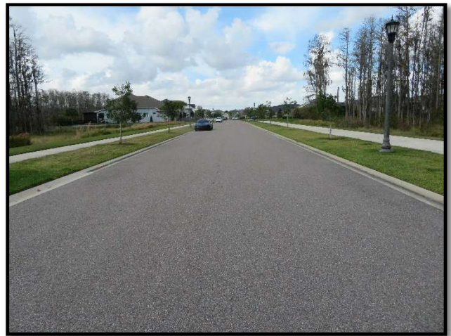
Asphalt pavement at Aviles Parkway
