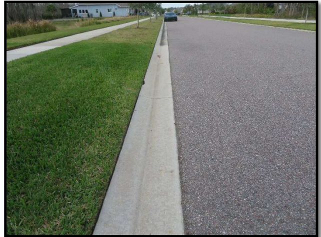
Concrete gutter overview
