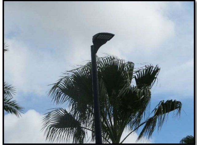
Light pole and fixture at pool
