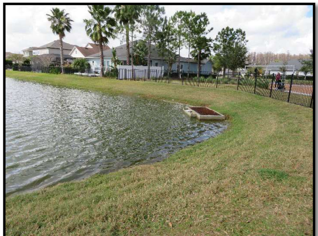
Pond shoreline and outlet structure
