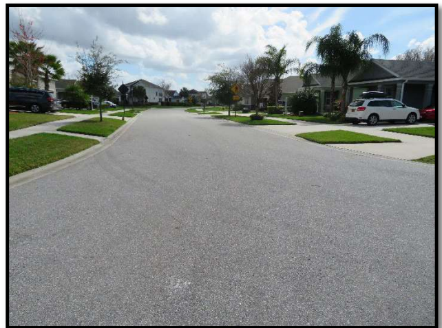
Asphalt pavement at Trails Edge Boulevard
