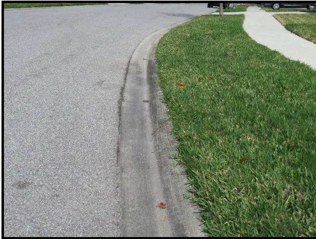
Concrete gutter overview
