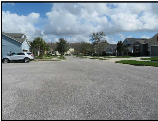
Asphalt pavement at Verona Lane
