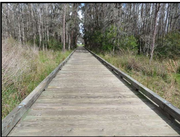
Boardwalk through natural preservation area
