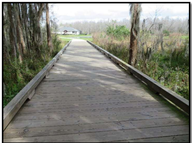
Boardwalk through natural preservation area
