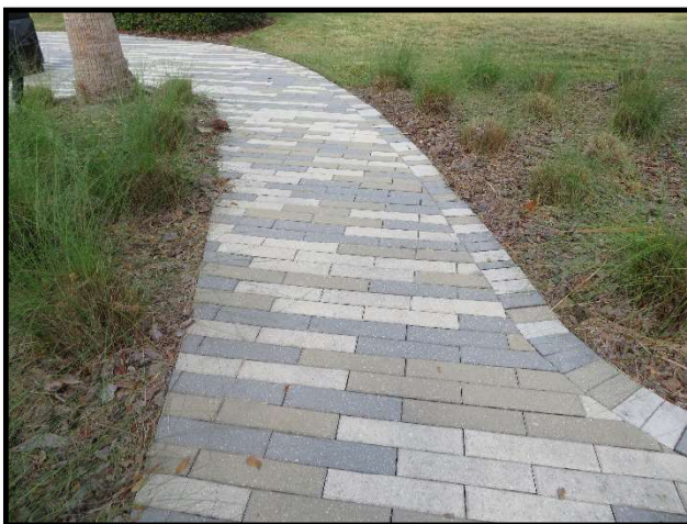
Masonry paver pool deck
