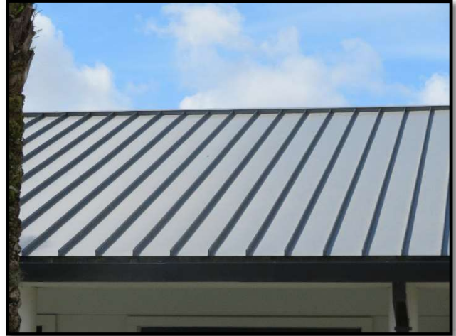
Clubhouse metal roof
