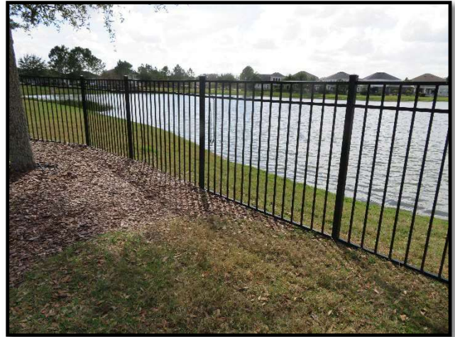
Aluminum fence adjacent to playground
